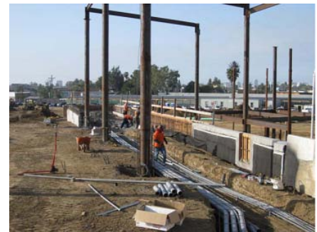
Backfill at Building A Retaining Wall
